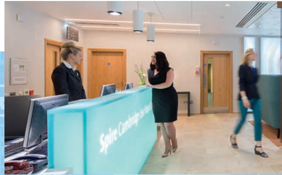
Additional Dali control supplied for an existing illuminated reception counter, allowing this to also link to the BMS
